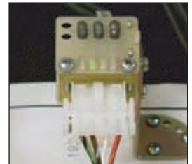
Blinking LEDs indicate wire routing.
